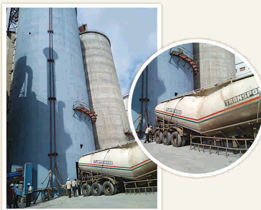
Converted Cement Silo to Fly Ash Silo
